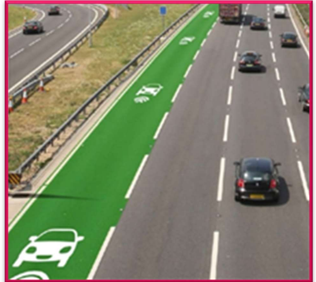
Figure 39: Wireless in road charging
